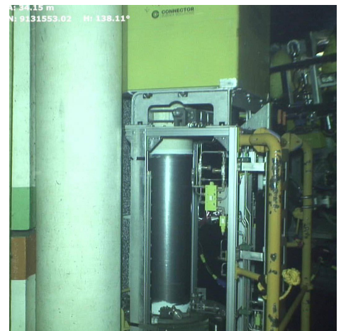
03 // CSS coating removal operation
