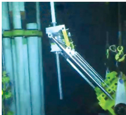
02 // Mounting of CSS connector installation frame
