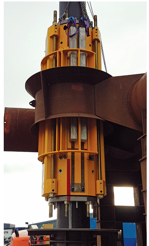
05 // Conductor clamp system integration test complete
