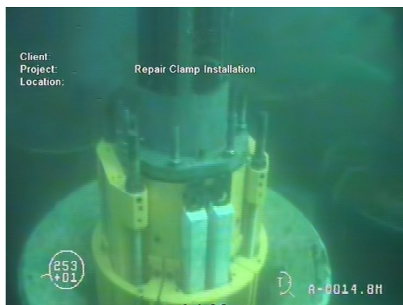
04 // Conductor repair clamp installed
